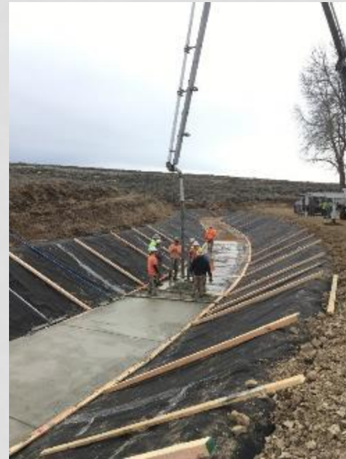
Kittitas Reclamation District South Branch Canal lining
